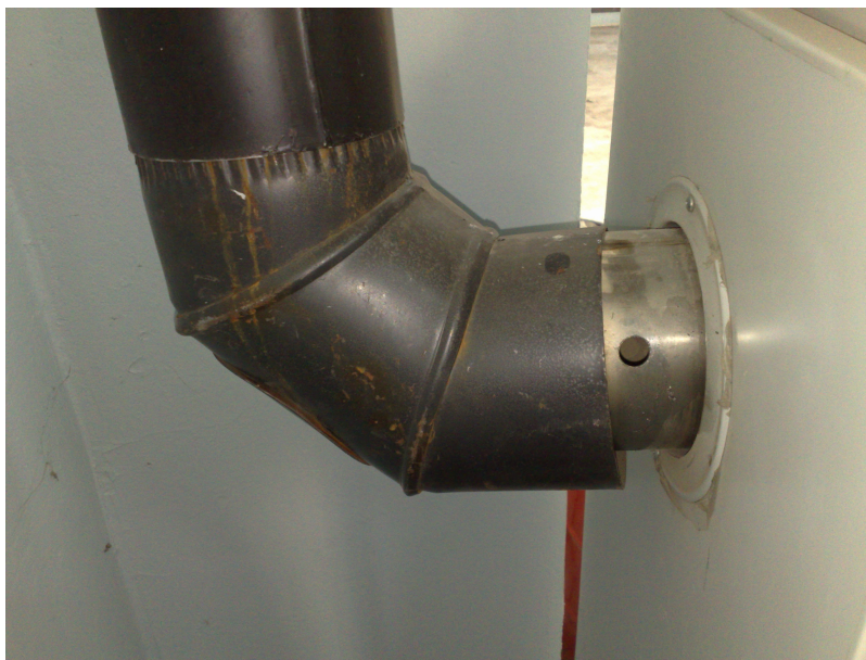
Picture 4. Measuring place on ventilation duct of boiler, type “B23”, manufacturer “GENERATORE D’ARIA LALDA”
